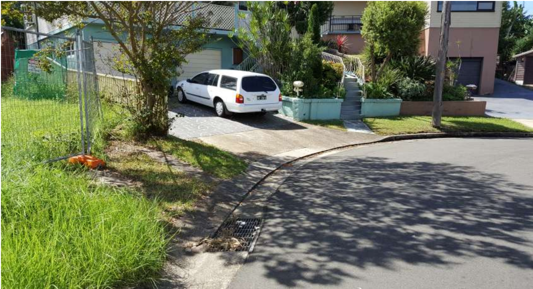
Figure 5 – Existing butterfly grate on Links Ave (Sourced: 06/04/2017)
